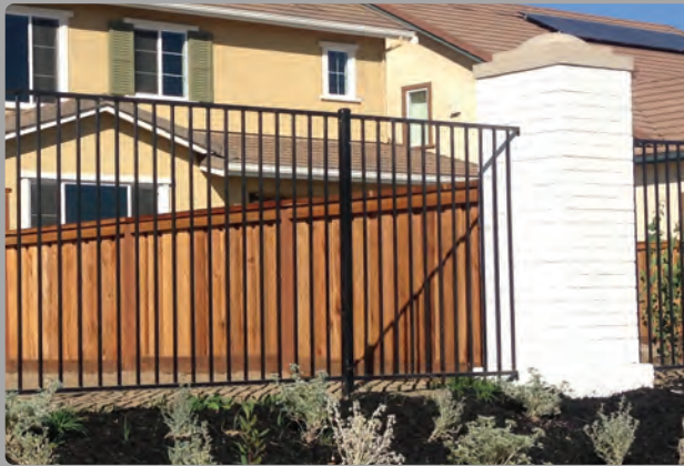
8' Tall Masonry Column with Open View Fence (5' Tall Tubular Steel Fence @ Linear Park & Lake Frontage)
