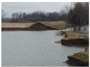
Figure 6.2 and 6.3, Levee breaches along the Wabash River
