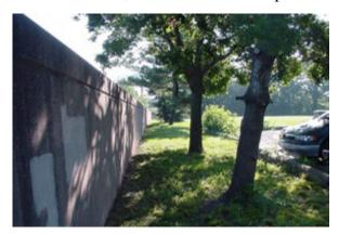
**Figure 2.51** *UNACCEPTABLE. Trees growing too close to floodwall. (KY)*
