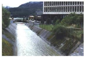
**Figure 2.74** *ACCEPTABLE* concrete lined channel. (AK)
