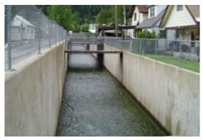
**Figure 2.72** ACCEPTABLE concrete lined flood control channel. (ID)
