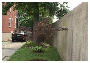
**Figure 2.52** UNACCEPTABLE. Trees growing too close to floodwall. (KY)
