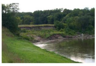
Figure 2.15 UNACCEPTABLE. Slope failure and Figure 2.16 UNACCEPTABLE. Slope failure and erosion caused by inadequate channel bottom and erosion on a channel improvement project. (MN) side slope protection. This was a direct result of bottom scouring that undercut the levee slope and erosion caused by turbulent flow at the end of the bank protection. (ND)
