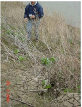
**Figure 2.34** UNACCEPTABLE cracking with landside pooling, Whitehead Levee Project, (IA)
