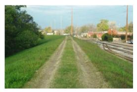
**Figure 2.39** *UNACCEPTABLE rutting in levee.* (OK)
