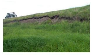
Figure 2.17 UNACCEPTABLE earthen embankment failure.~(MN)
