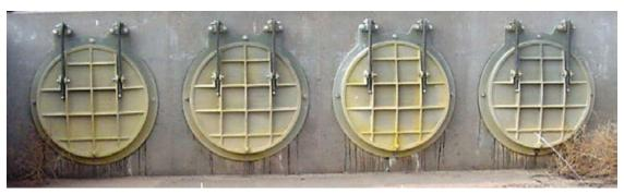
Figure 2.64 ACCEPTABLE flap gates in earthen levee. (KS)
