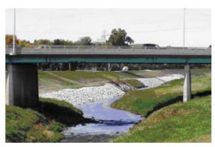
**Figure 2.26** ACCEPTABLE riprap for erosion control. (NE)
