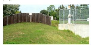
**Figure 2.11** *UNACCEPTABLE* encroachment. Residential and rural fences crossing the levee. (ND)
