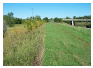
**Figure 2.32** UNACCEPTABLE long grasses and trees on levee side slopes. (ND)
