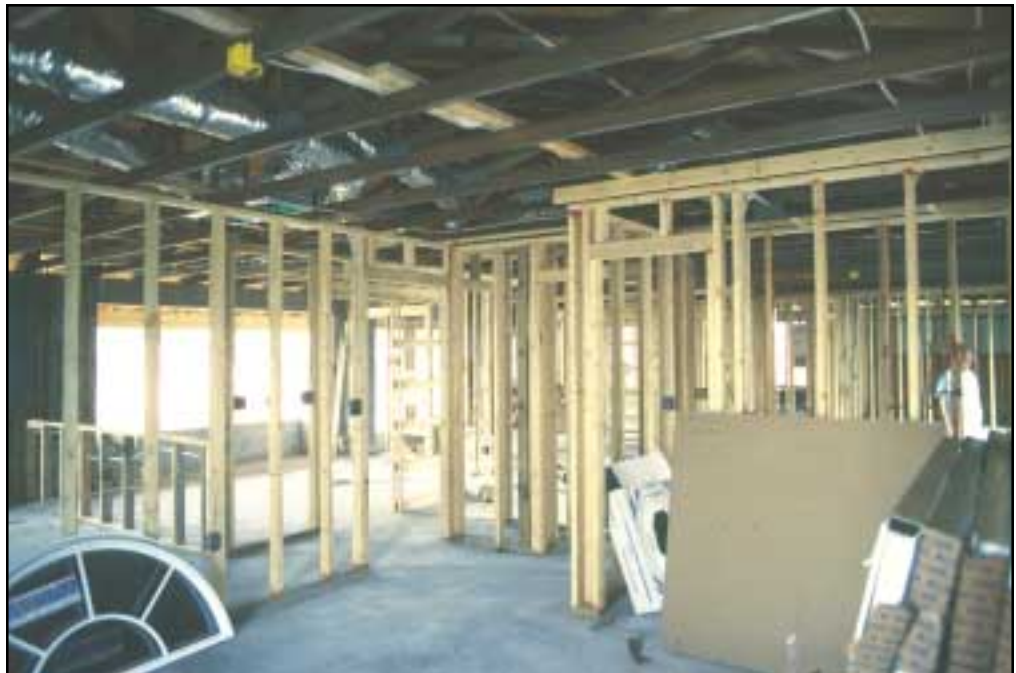
Figure 30 Interior partition walls and utilities are added.
