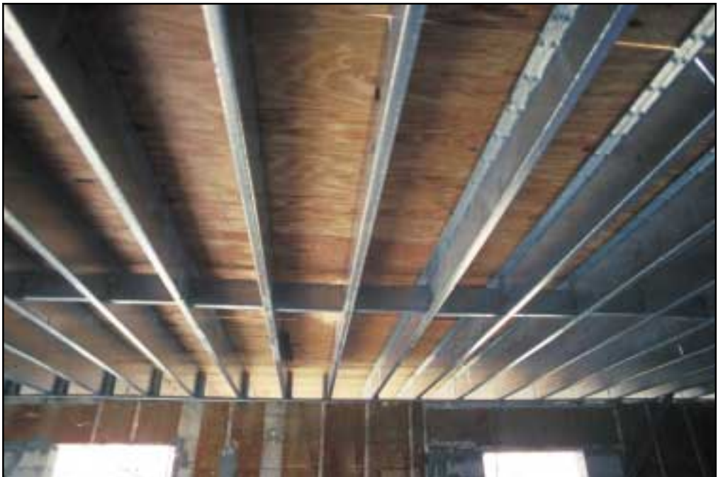
Figure 55 Metal framing also supports the floor of the new second story.
