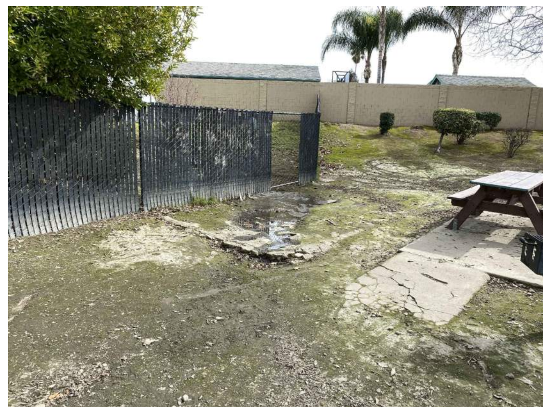
Existing storm drainage outfall at the northeast corner
